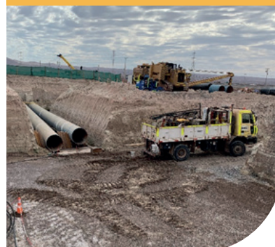
Technical Work Inspection for the Project: "Construction of Collector Pit and Drainage Pool for the Copper Concentrate and Desalinated Water Transportation System (Pipeline)", located at Junction under Route 5. Customer Teck QB2.
