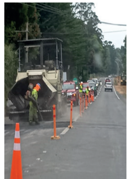
Replacement of wearing course of asphalt concrete crossing Route 126 S (Coelemu)
