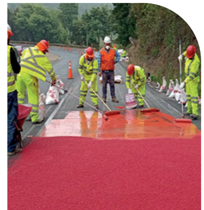
High friction seal junction Route 126 S (Coelemu) - Junction 0-274 (Tomé)
