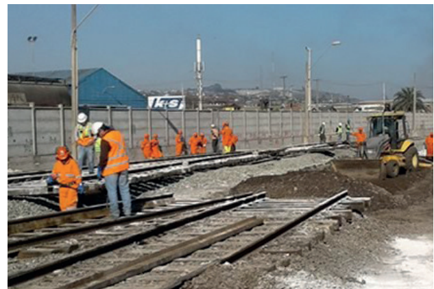
Spill of sulfuric acid on the railway infrastructure to the inside the terquim unloading terminal land.
