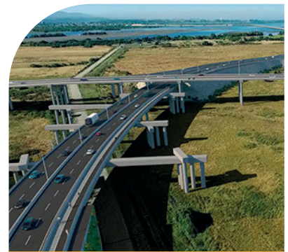
Industrial bridge concession project
