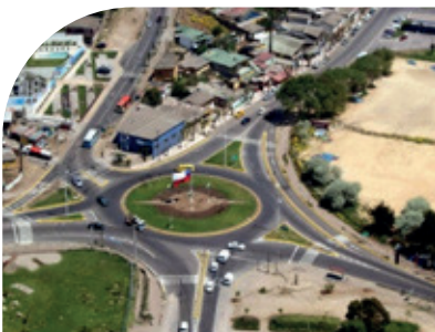
Improvement of route F-30, cemetery sector Concón – Concón roundabout
